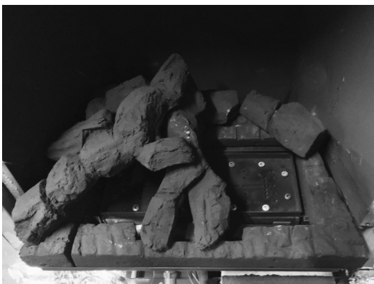
Left The coal flake sits to the left between bottom left coal piece and side piece
