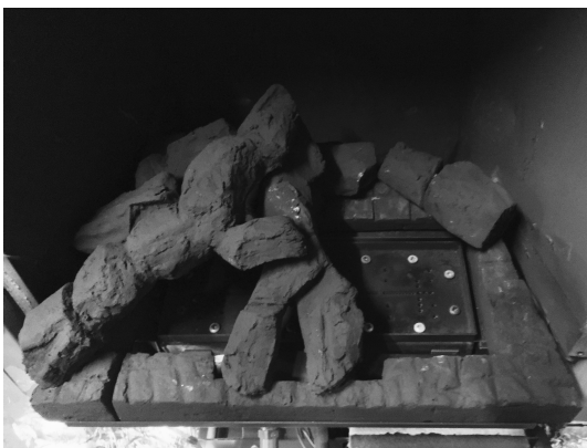
Left The coal flake sits to the left between bottom left coal piece and side piece
