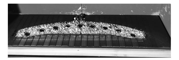
The fire base is placed into position ensuring the pilot is not fouled ,the base pushes down into place ,it is a tight fit and if need be push back towards fibre back to get it in place
